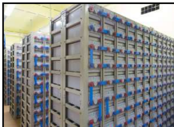
Traditionally, battery modules have been connected by front bus-bars or jumper cables.
